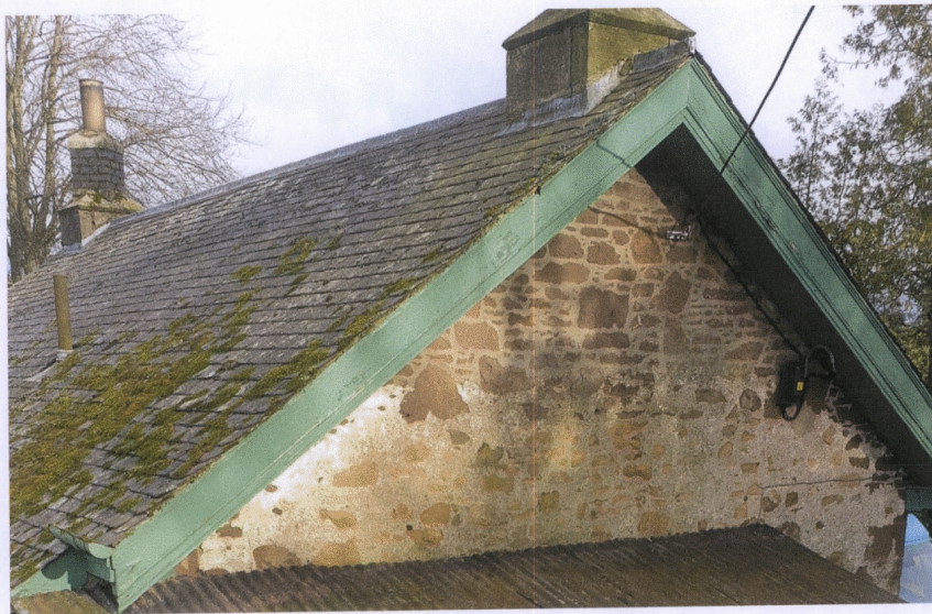
Picture 6: - Clearly visible area where West gable wall head has previously been raised
