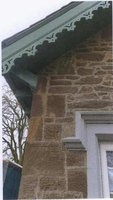
Picture 8: - Corner stones have been raised
