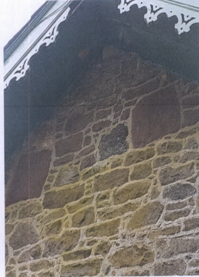
Picture 5: - Area where east gable wall head has been raised
